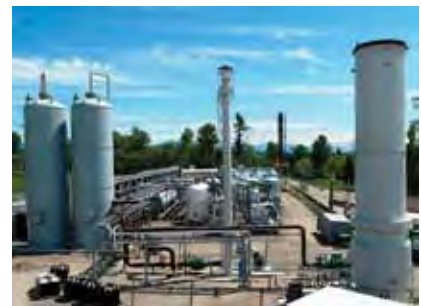
Cedar Hills Bio-Energy Facility in Maple Valley, WA
