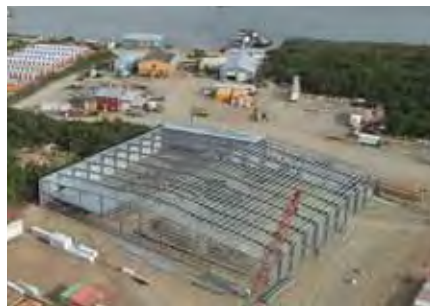
Salmon processing plant under construction in Naknek, AK
